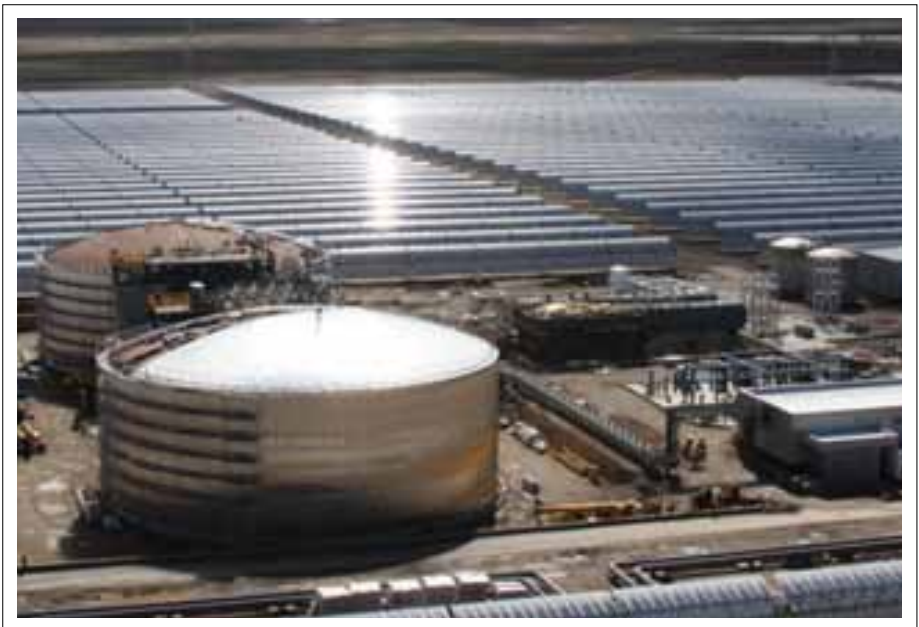
Plate 1: Two thermal storage tanks and field at Andasol Plant (Source: Solar Millennium)
