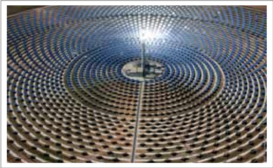
Plate 2: Aerial view of Gemasolar plant in operation ( Source: www.torresolenergy.com, Image library )
